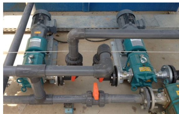
Rotary Lobe Type Permeate/Backwash Pump
