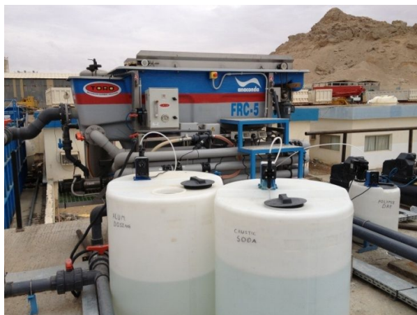
DAF System with Dosing Pumps
