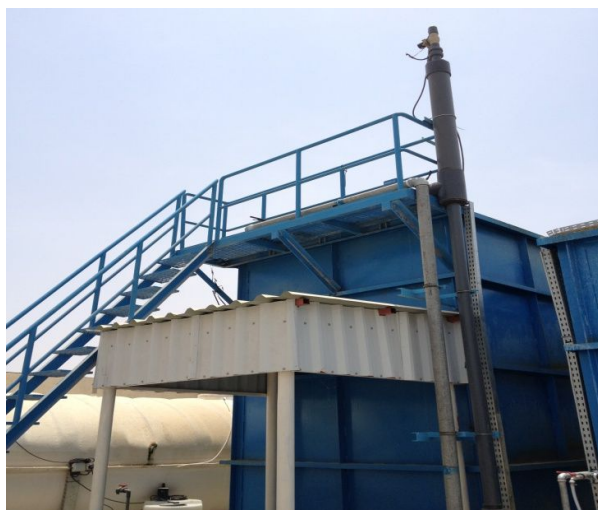
MBR Tank with Degassing Vessel
