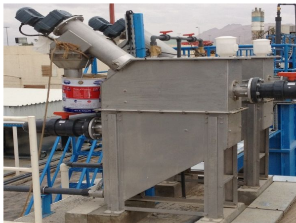
Fine Screen with Grit Removal System
