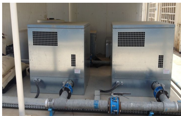
Aeration Positive Displacement Blowers
