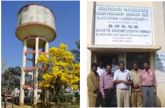
BWSSB Overhead Tank, Office & Staff
