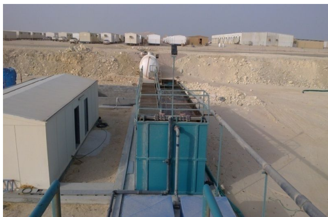
Top View of STP showing Blowers, Aeration Tanks, Control Panel & Operations Room
