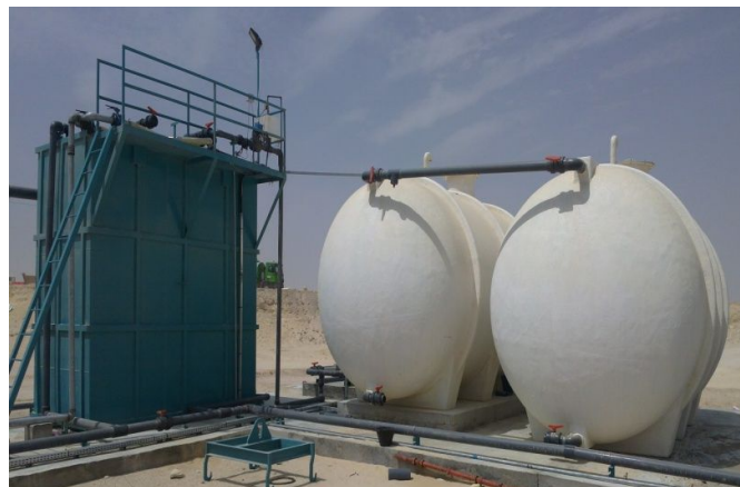
MBR Tank and TSE Tanks of STP
