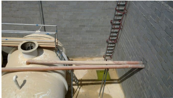
Equalization Tank of STP
