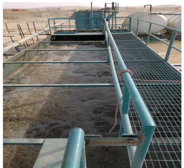
Anoxic/Aeration/Nitrification MSEP Tank
