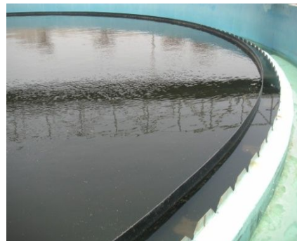
Settling Tanks with TSE
