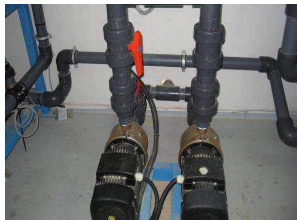
UF System Feed Pumps
