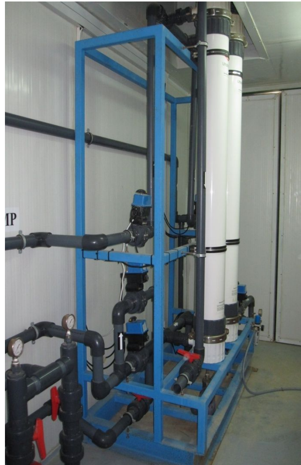
UF Module inside a 40 feet container in Duqm, Oman
