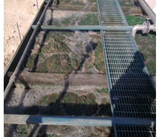
Top View of MBBR-IFAS Tank with MBBR Bio Media
