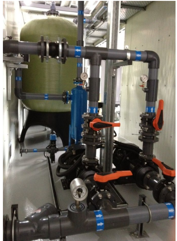
Multi Media Filter in RO Plant
