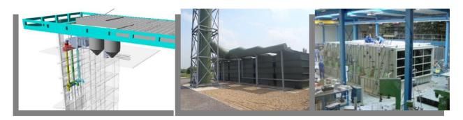
**China -** Refurbishment and upgrade of a biofilter treating 160,000 m3/h->60°C odorous air of a Nutreco Shiha Zuhai Fish Feed factory.
