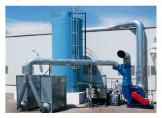
**Rumania** – Vocus (trickling) system at Multipack, a flexographic printing company. Biological treatment of high concentrations of ethanol, ethyl acetate and other VOC's in 1 tower. 6000 m<sup>3</sup>/h with 50 ton VOC/year
