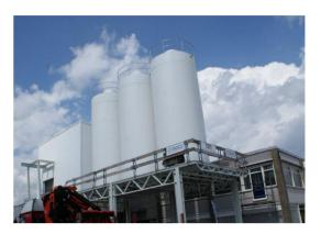
**The Netherlands** – Vocus (trickling) system at Altacel Transparant, a flexographic printing company. Biological treatment of high concentrations of ethanol, ethyl **acetate** and other VOC's in 3 towers. 9.500 m<sup>3</sup>/h with 100 ton VOC/year
