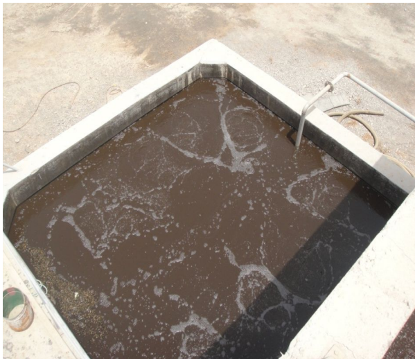
Good Quality MLSS inside Aeration Tank
