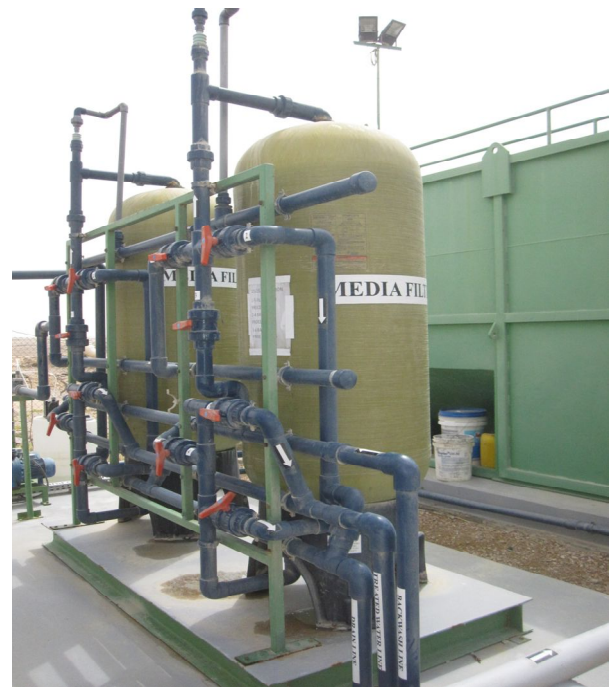
Filtration System of ASP STP
