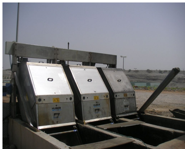
Mechanical Fine Screen, 6 mm
