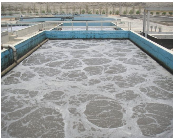
Aeration Tank With Fine Bubble Diffusers
