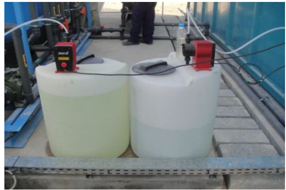
Hypochlorite Dosing System for Disinfection
