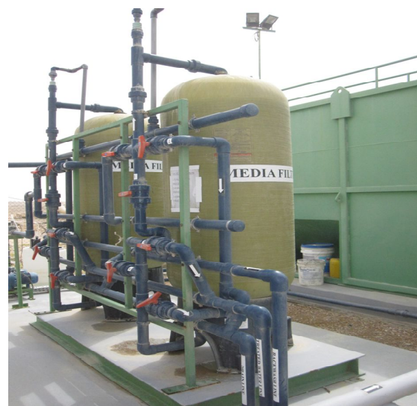
Filtration System of MBBR STP
