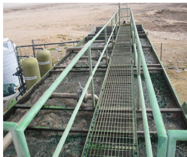
Aeration Tank filled with Bio Media
