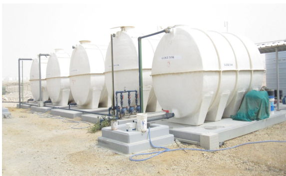
Equalization/Sludge Tank with Raw Sewage Pumps
