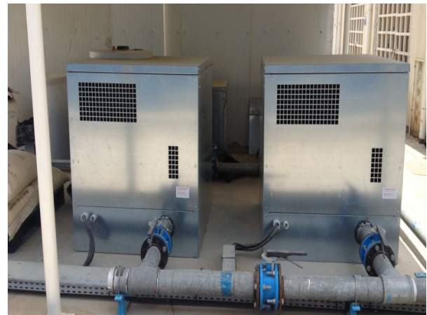
Aeration Positive Displacement Blowers
