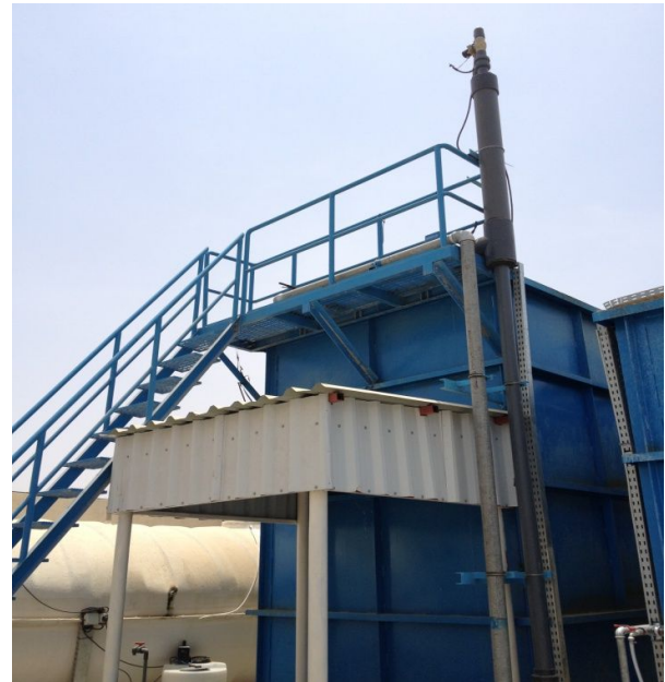
MBR Tank with Degassing Vessel
