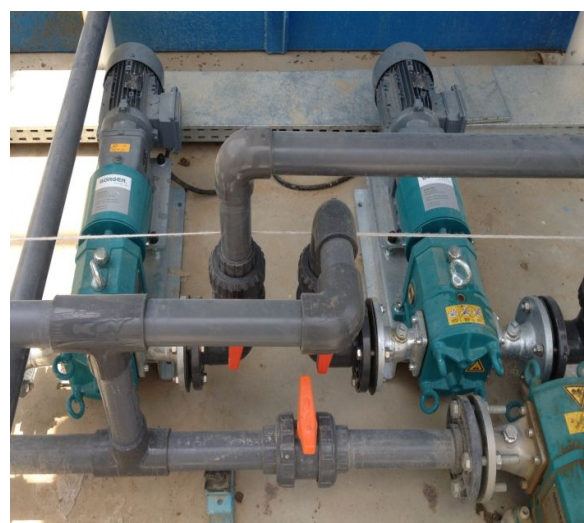
Rotary Lobe Type Permeate/Backwash Pump
