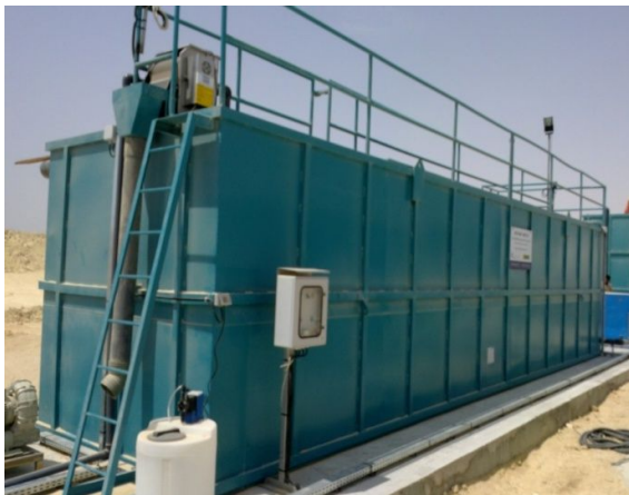
Containerized MBR Technology WTP
