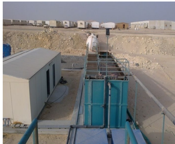
Top View of STP showing Blowers, Aeration Tanks, Control Panel & Operations Room
