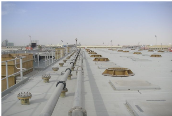
Gas Piping at Ajman STP UASB Reactor
