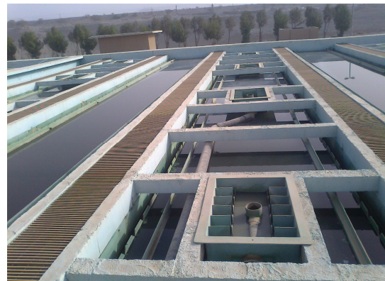
Feed Inlet Box of UASB Reactor at RAK STP
