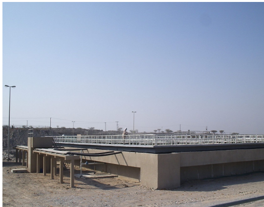
UASB Reactors of 40 MLD STP at RAK, UAE
