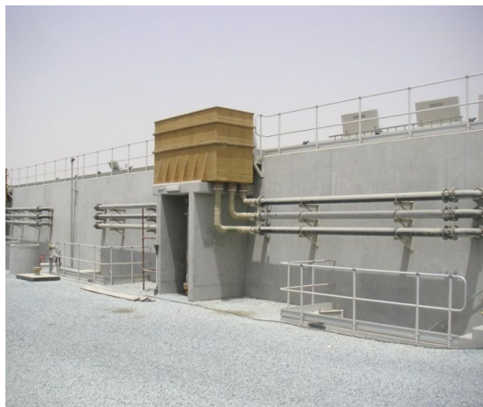
UASB Reactors of 49 MLD STP at AJMAN, UAE
