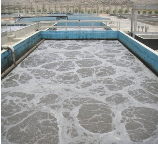
Aeration Tank with Fine Bubble Diffusers
